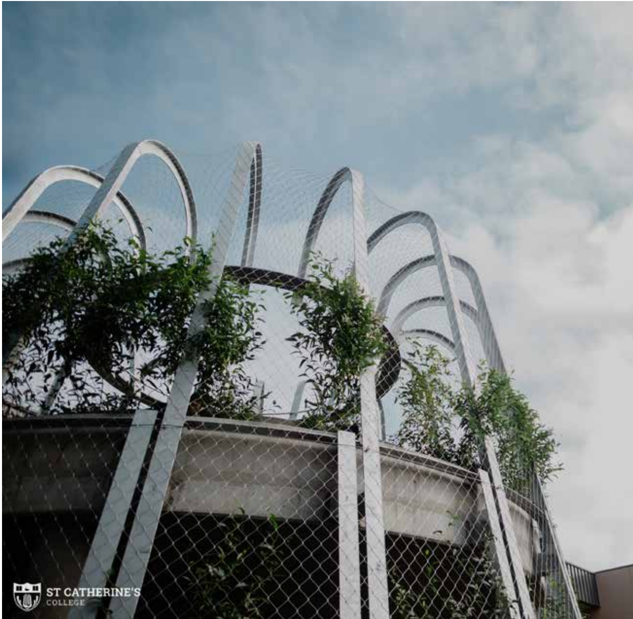
The central feature of the building is 'the banksia' that has on its top level a smoking ceremonial space for indigenous students. Eventually, flowering vines will cover the trellis.
