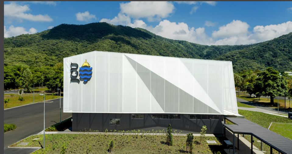
The form of the building is at the scale of the Kuranda National Park range that overlooks the JCU site.
