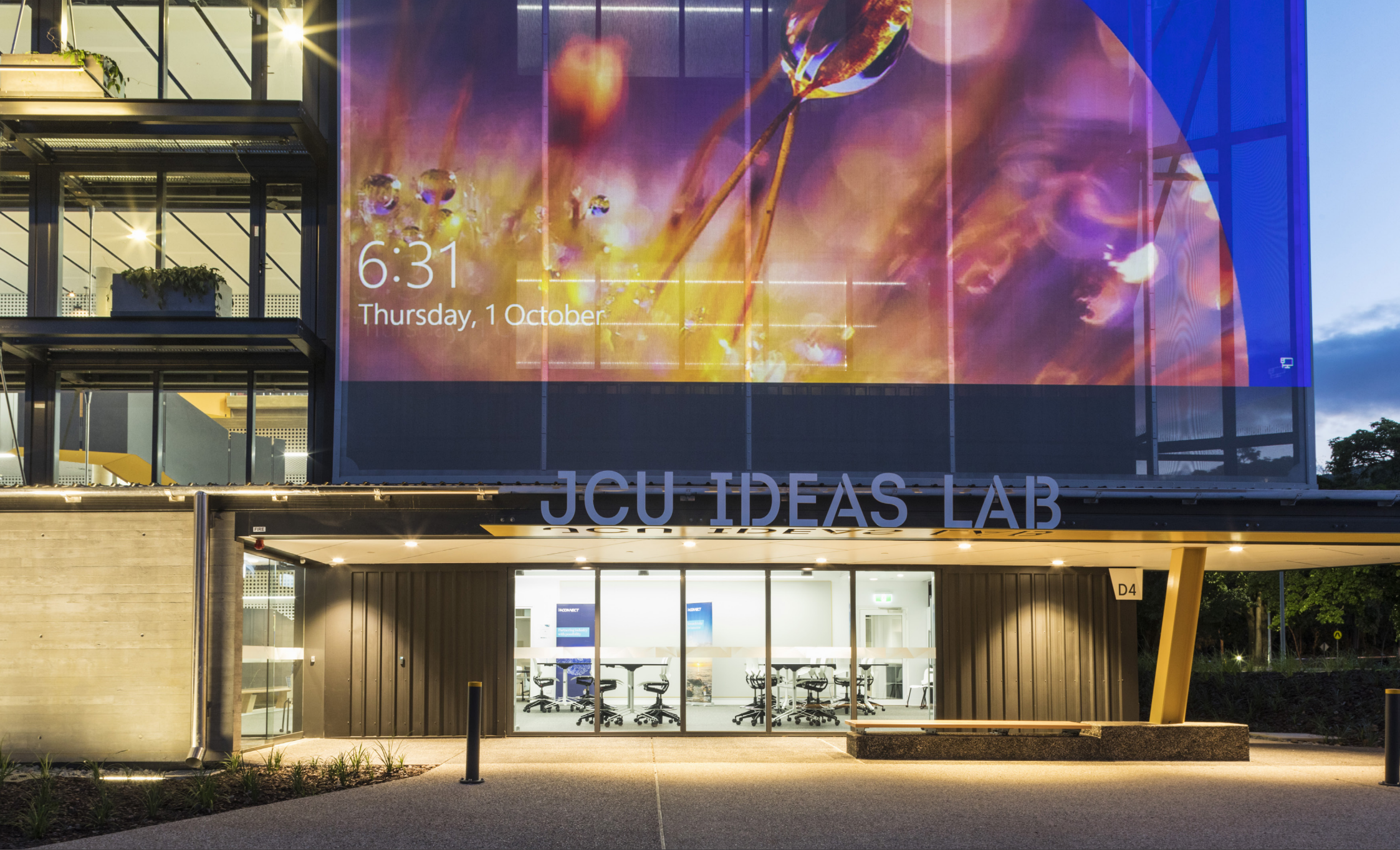
Large format projectors cast images onto the screen at night further animating the facade to become a beacon in the landscape for the University.
