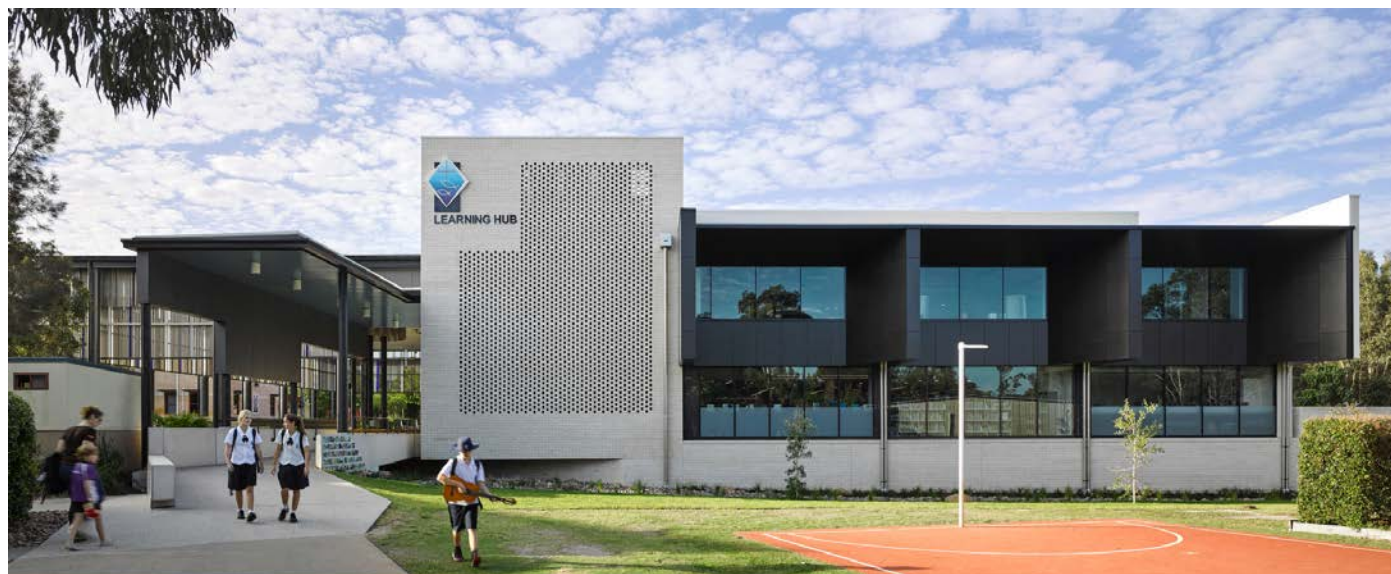
The new Learning Hub, at the centre of the campus, has set up the strategy and sequence for future construction stages.
